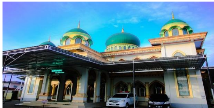
Figure 8. Assembly ambulance in the mosque
