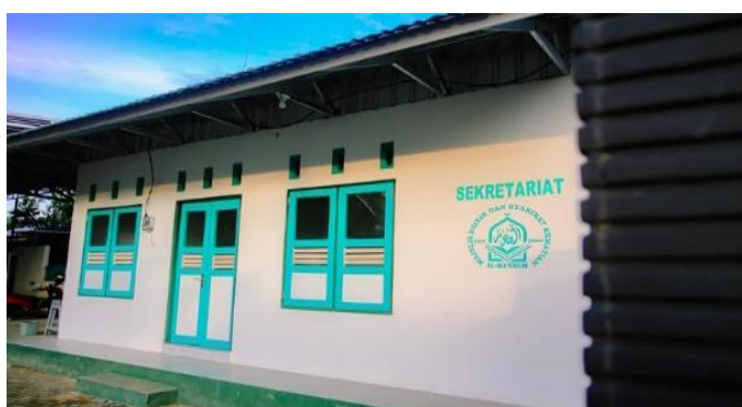
Figure 3. The office of the management of the Dhikr Assembly and Funeral Society
