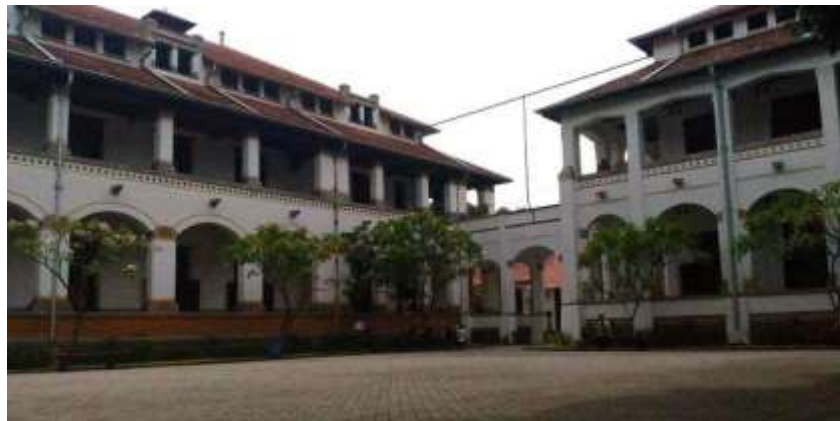
Picture 3 The building of Lawang Sewu
