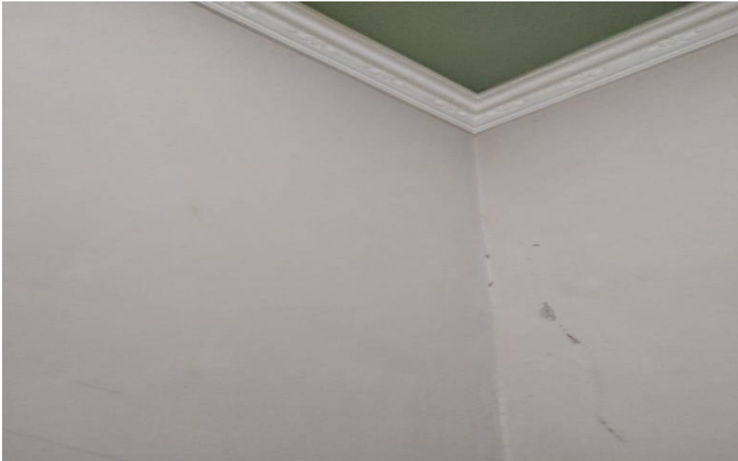
Figure2. Photographs of empty wall
